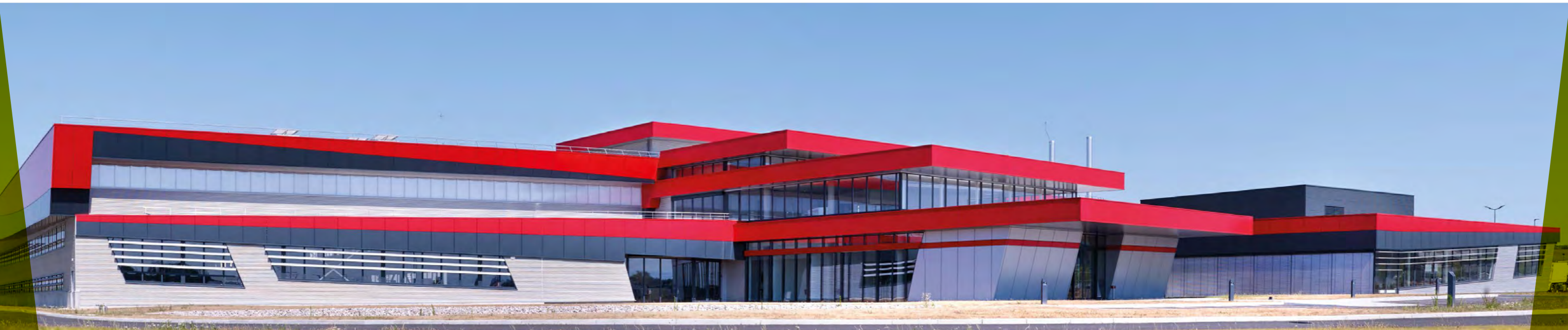
■ Facade, Danpatherm K7 12 and 16, 900 mm, clear Softlite, 2,350 m 2
