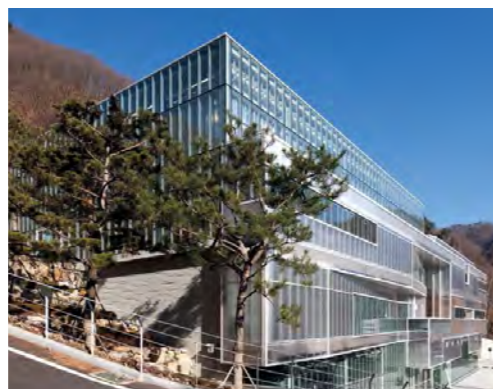
■ Facade and roofing, Danpalon® 12, 900 mm, clear, Danpalon® 10, 600 mm, ice, 3,500 m²
