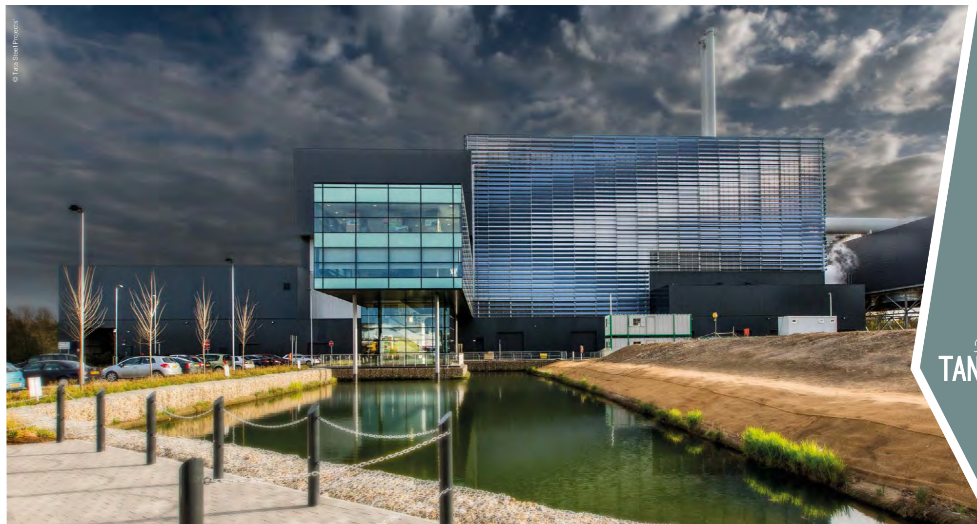
■ Facade, Danpalon® 16, 1,040 mm, Ice Softlite, 13,896 m²
