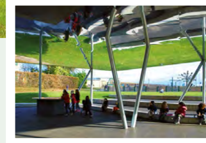
■ Ventilated Rainscreen, Danpalon® BRV 12, 600 mm, clear with iridescent gold, with adhesive tape, 160 m 2
